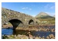
The photogenic Sligachan Old Bridge over the Sligachan River on the Isle of Skye is close to the A87 linking Broadford and Portree, just past the end of Loch Sligachan. Engineer Thomas Telford built this bridge between 1810 and 1818. It has three arches with a hump over the central arch, a characteristic of bridges at that time.
